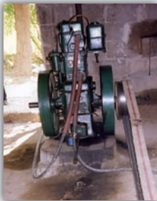
■ Photo 2. A water pump in Gaza
