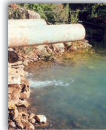
■ Photo 5. Water pipes at the Wazzani Springs in southern Lebanon
