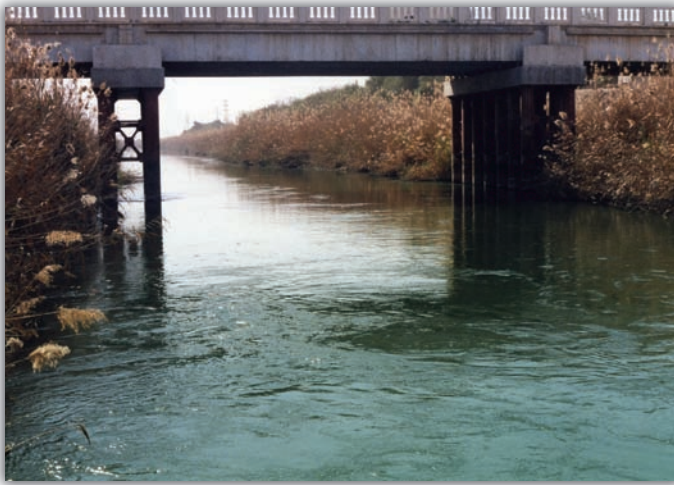
■ Photo 24. A manmade drainage channel for the Euphrates and the Tigris Rivers starting from west of Baghdad to the south designed with a projected average flow of 270 m 3 /s
