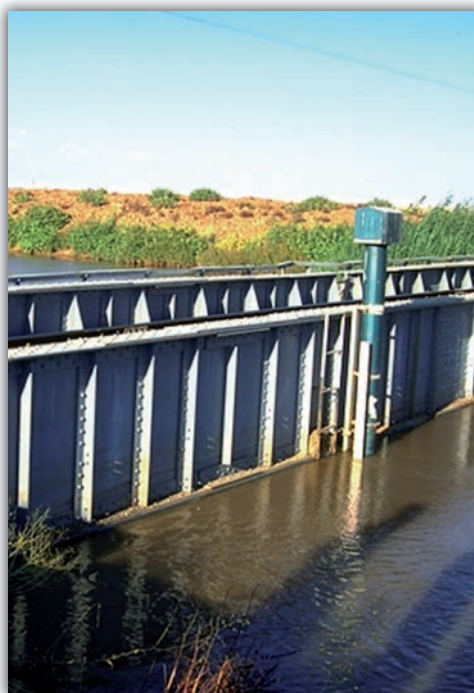
■ Photo 35. A railroad bridge with a water-measurement device over the Balih River on the Syrian side of the border with Turkey
