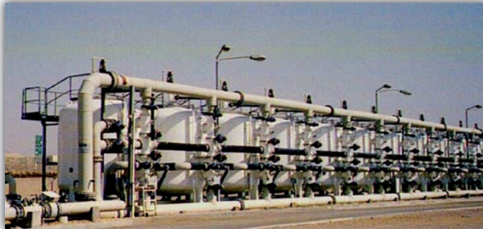
■ Photo 20. Desalination of brackish water is one part of the solution for both Parties
