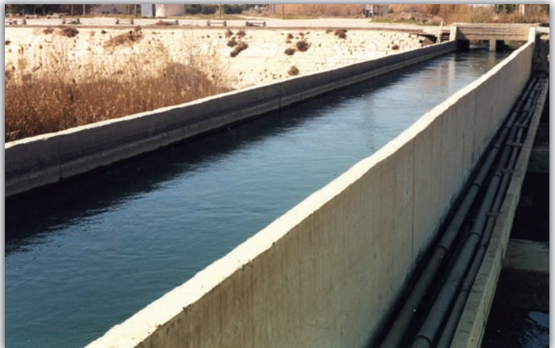
■ Photo 30. A culvert for an irrigation field from the Euphrates River south of Baghdad
