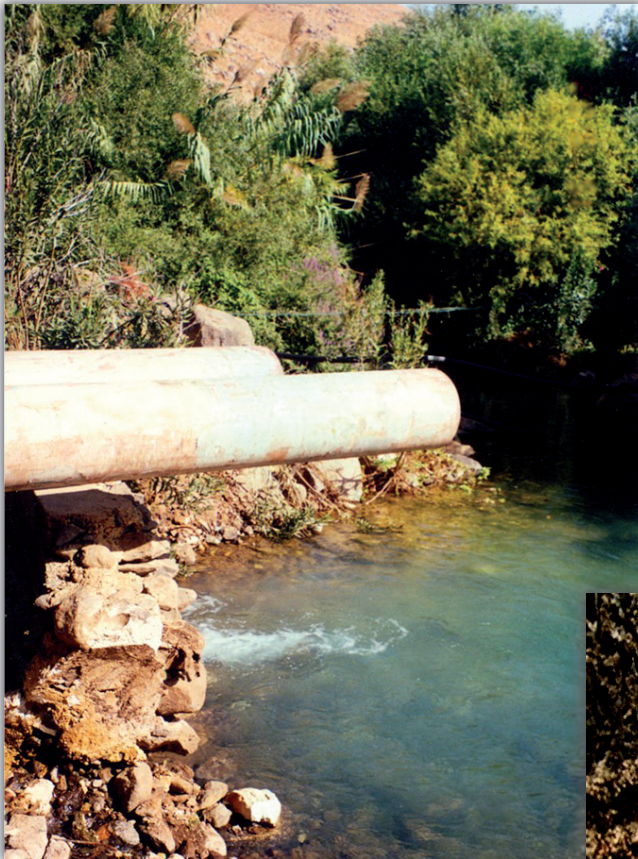
■ Photo 16. Water pipes at the Wazzani Springs in southern Lebanon
