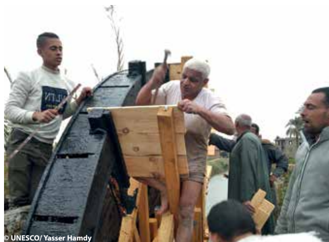
Image 24: Installing the waterwheel
