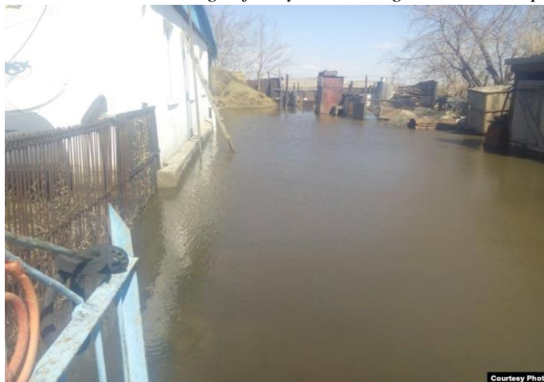
Figure 6.52. A flooded house in the village of Sarytobe, Karaganda oblast. April 17, 2017 247
