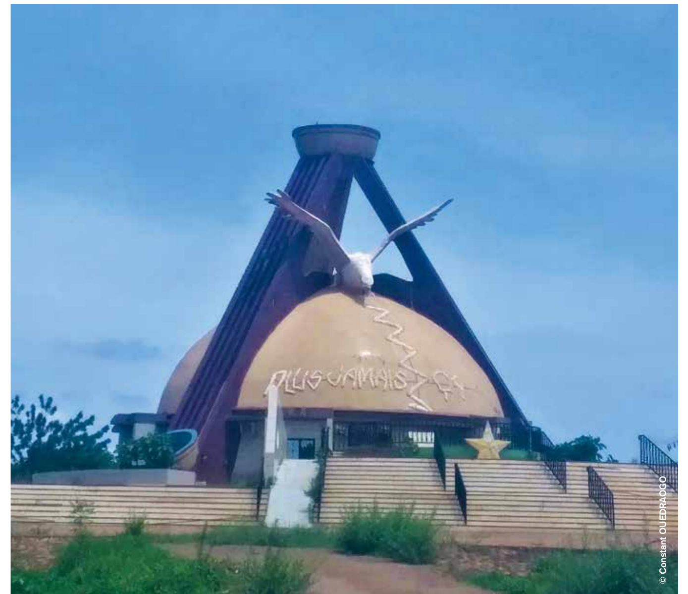
△ The Monument to the Martyrs in Ouagadougou, Burkina Faso, represents a broken calabash being sewed up by a dove that calls out with the phrase "never again!" The monument reminds that any repair always leaves indelible traces, just as forgiveness does not erase pain but reduces the reaction.
