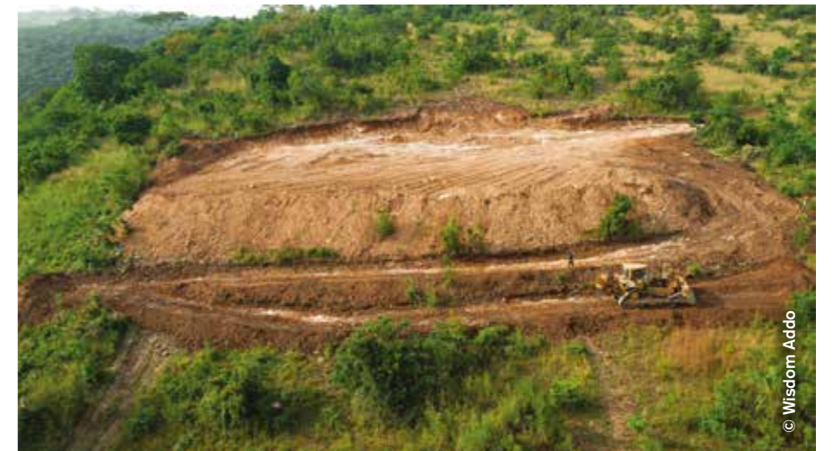
△ Clearing of the Peace Centre's site.
